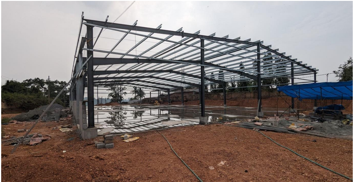
compressed bio gas plant construction in progress
