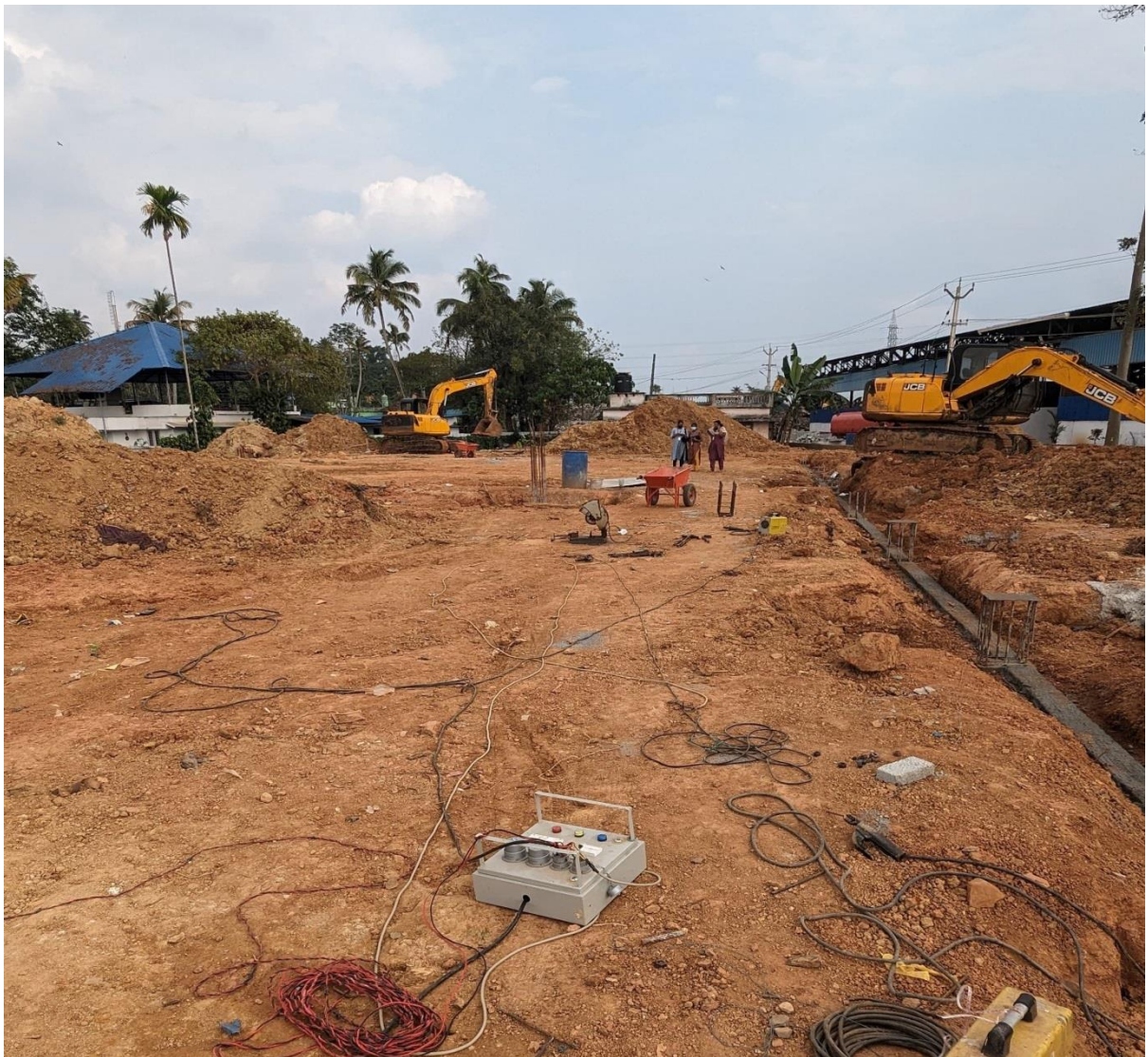
Preliminary construction work of BSF plant is being going on
