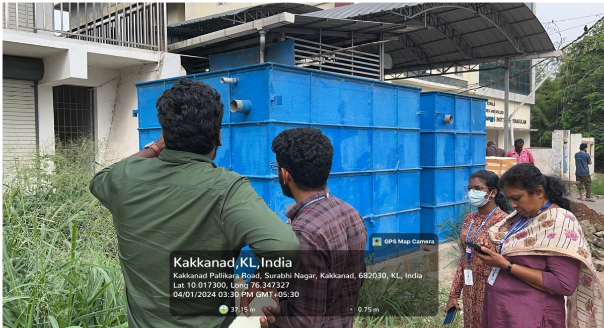
Ongoing construction of STP in Kakkanad Market
