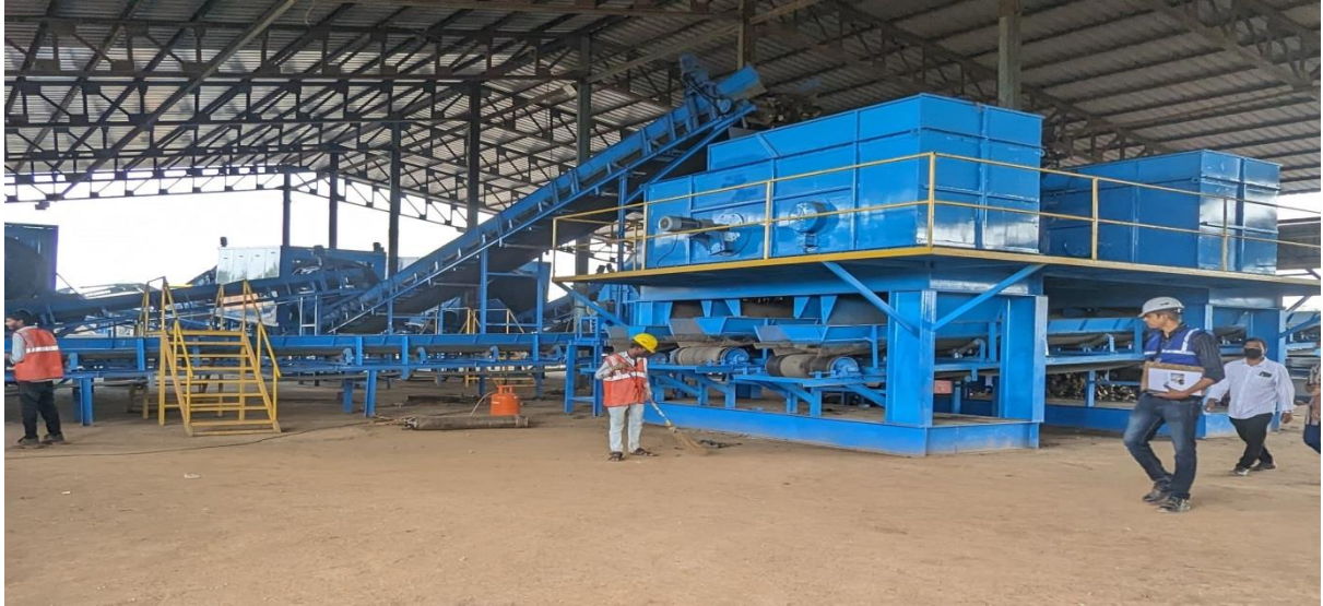
Trial run going on at Brahmapuram plant
